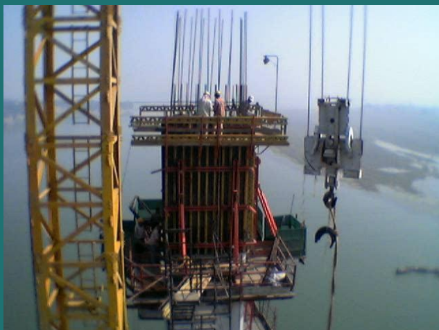
On-line health monitoring system for cable-stay bridge on Yamuna river
